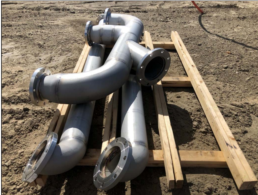
Fabricated steel piping for river and reservoir pumping structures.
