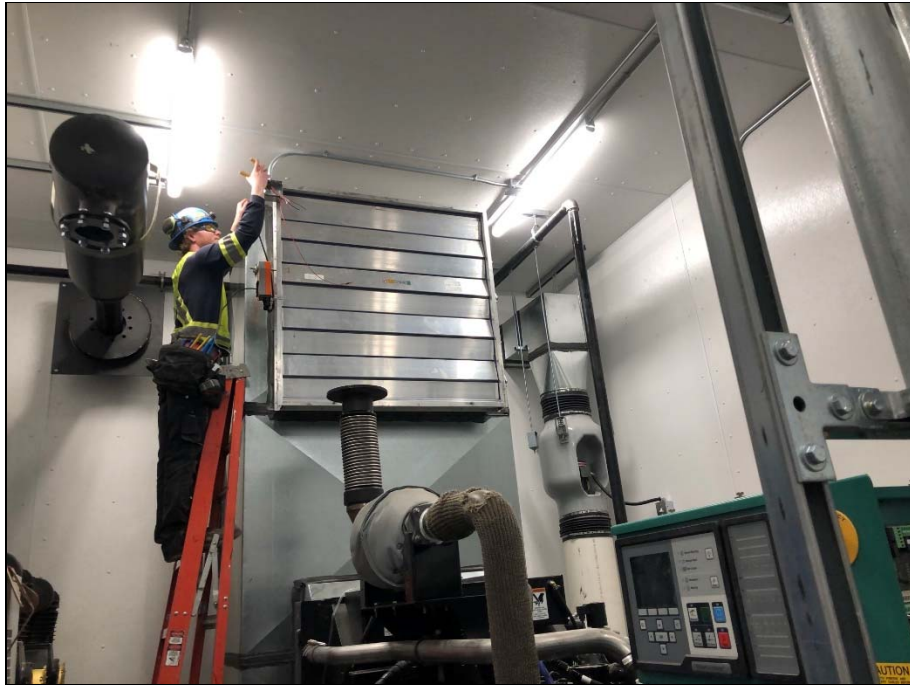
Generator room work underway.
