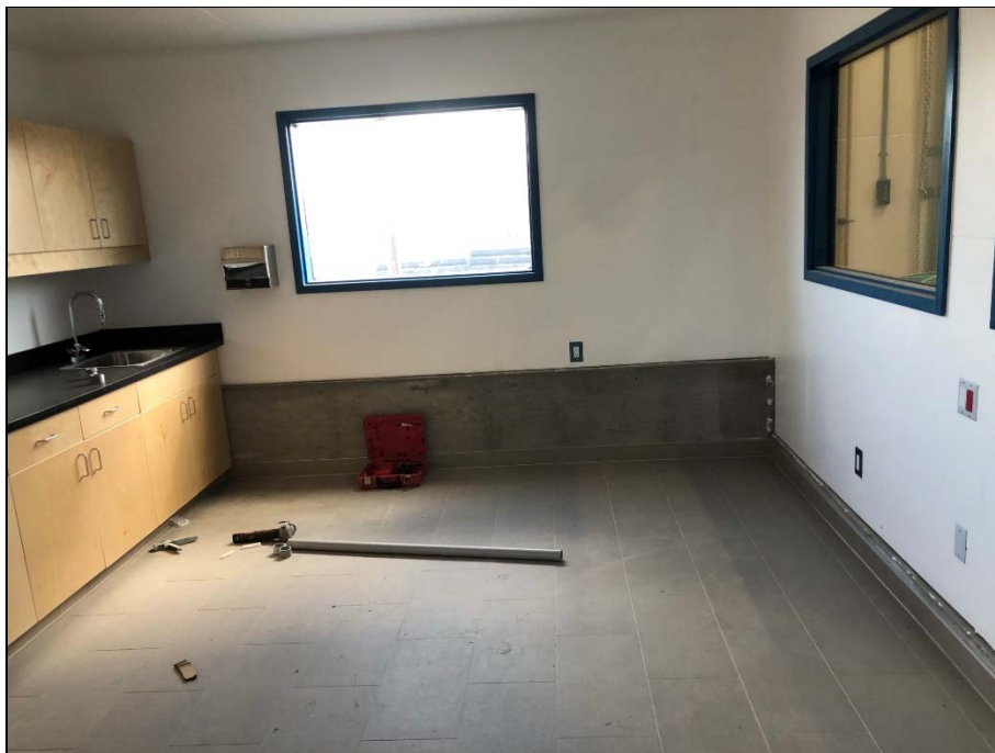
Office tiling complete.
