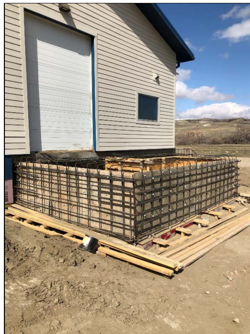
Loading dock rebar placement.
