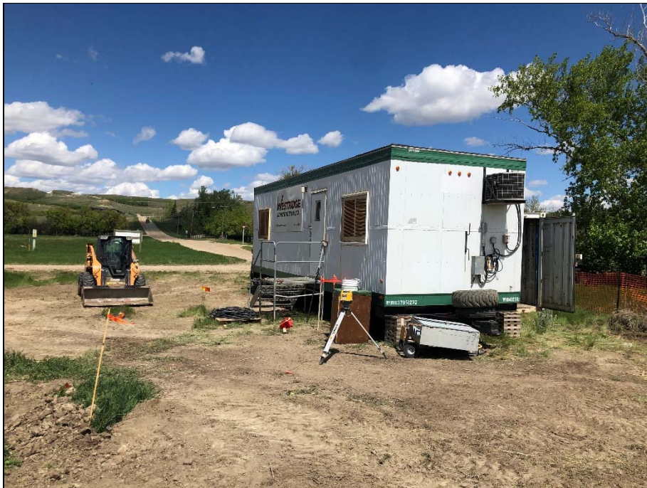
Westridge Construction site trailer and sea can on site.
