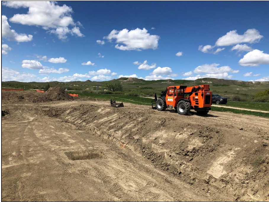
Water treatment plant excavation (looking northwest).
