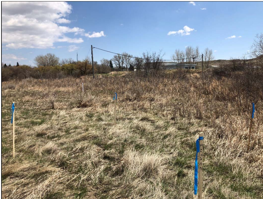
Location for raw water intake structure staked out.
