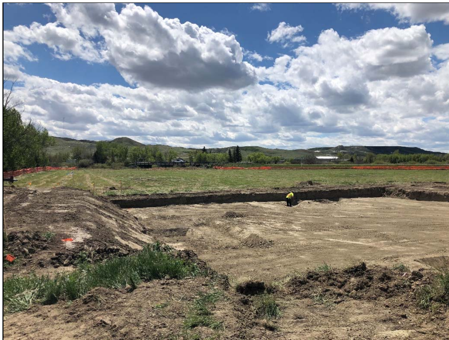
Excavation for water treatment plant base slab (looking south).
