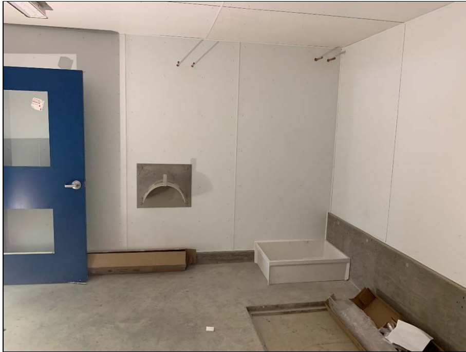
Chemical room FRP paneling in place.
