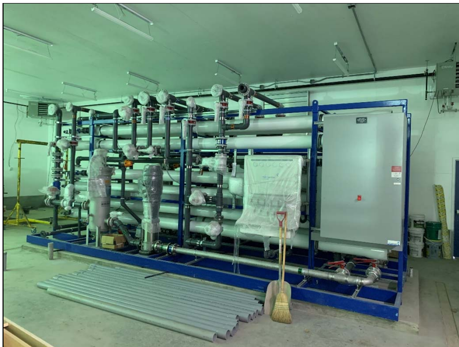
Nanofiltration (NF) skids were set in place but final placement required.
