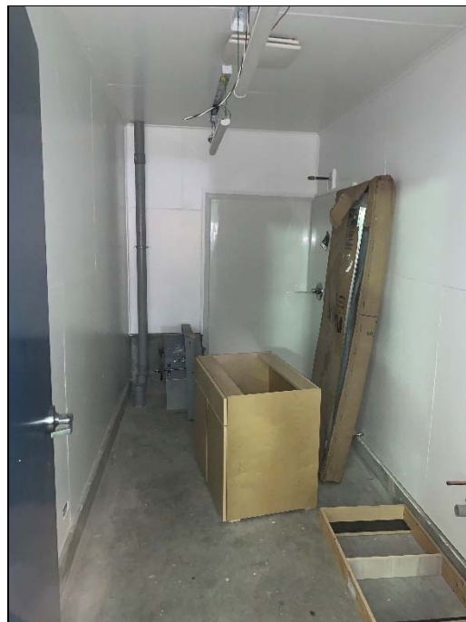
Washroom finishing underway.
