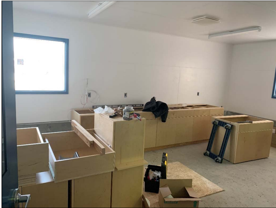
Office millwork on site; window installation underway.
