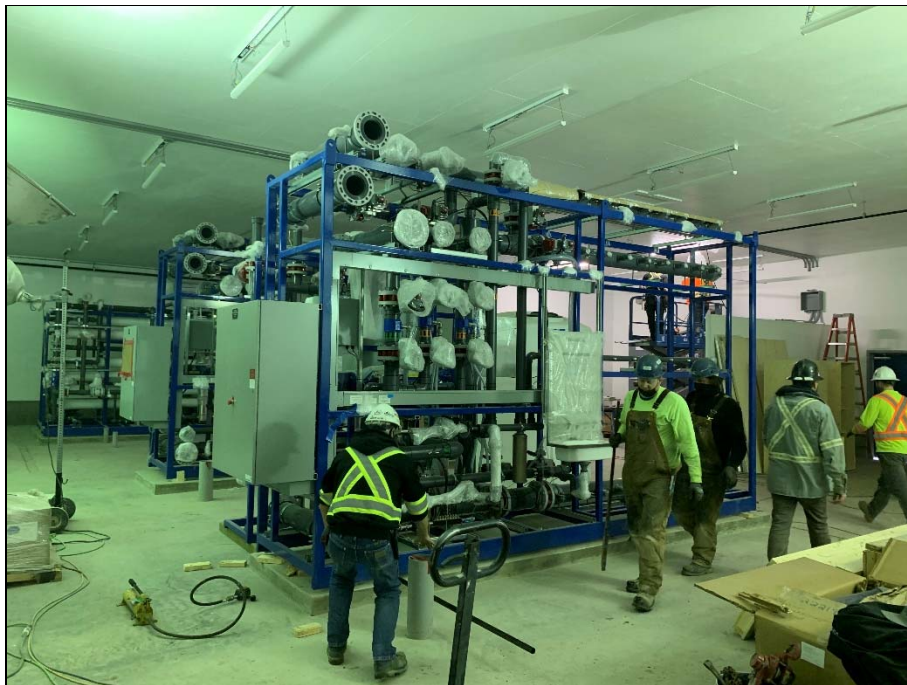
Treatment skids being moved into place.
