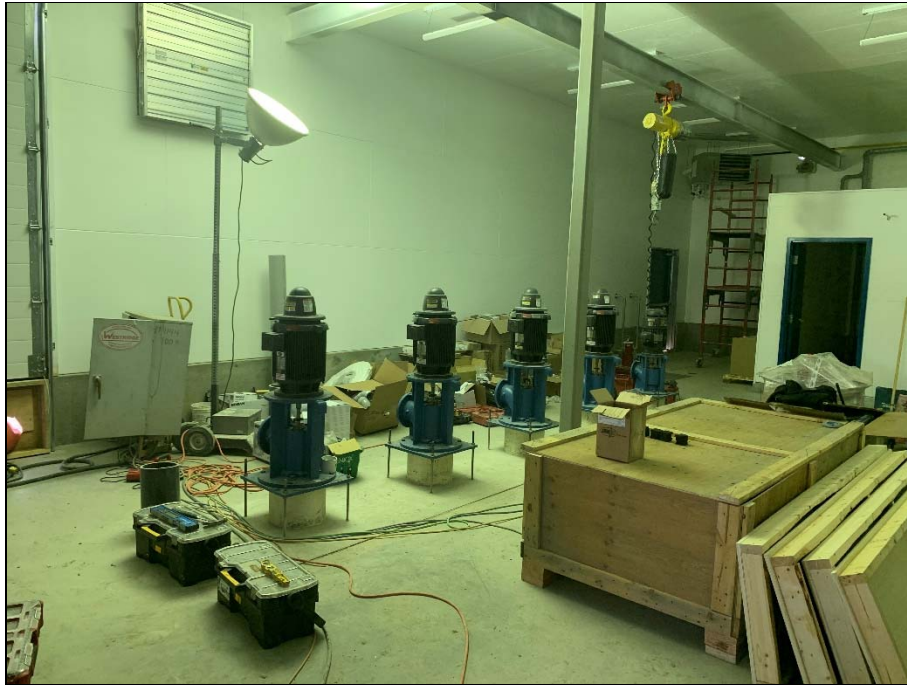
Distribution and truck fill pumps are set.
