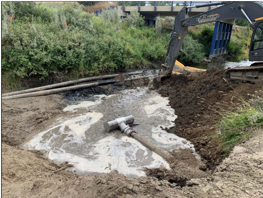
Removal of cofferdam to submerge intake structure.
