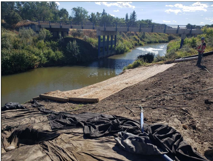
Riverbank vegetation restoration work underway.
