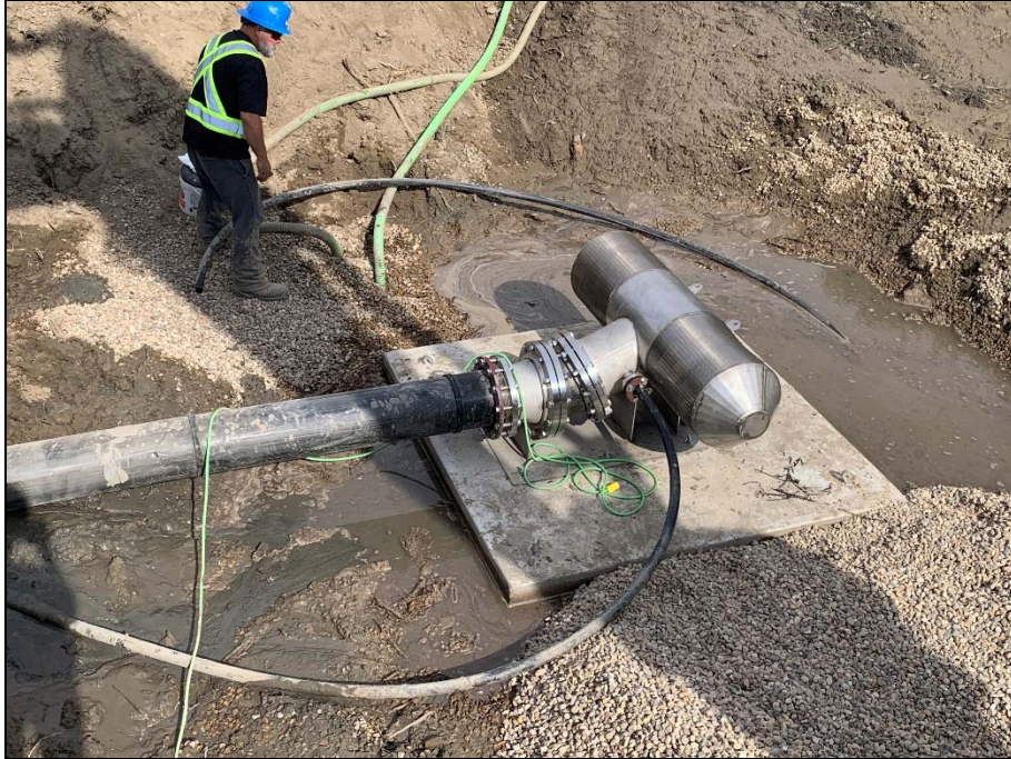
River intake and air scour line installation in riverbed.
