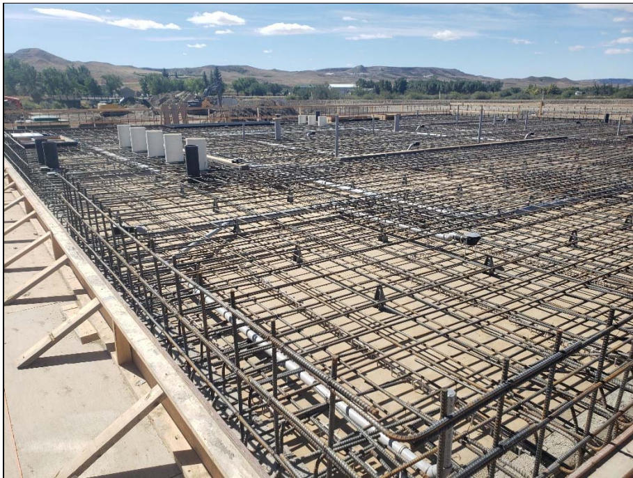
Top slab rebar and drainage piping inspection.
