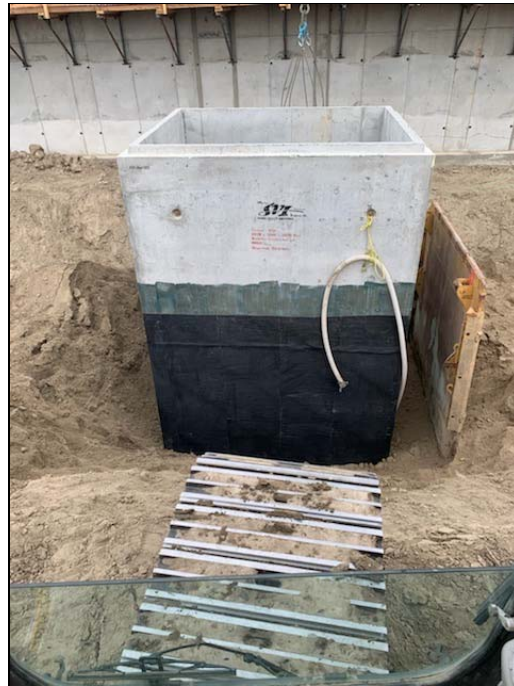
Reservoir intake structure installation.
