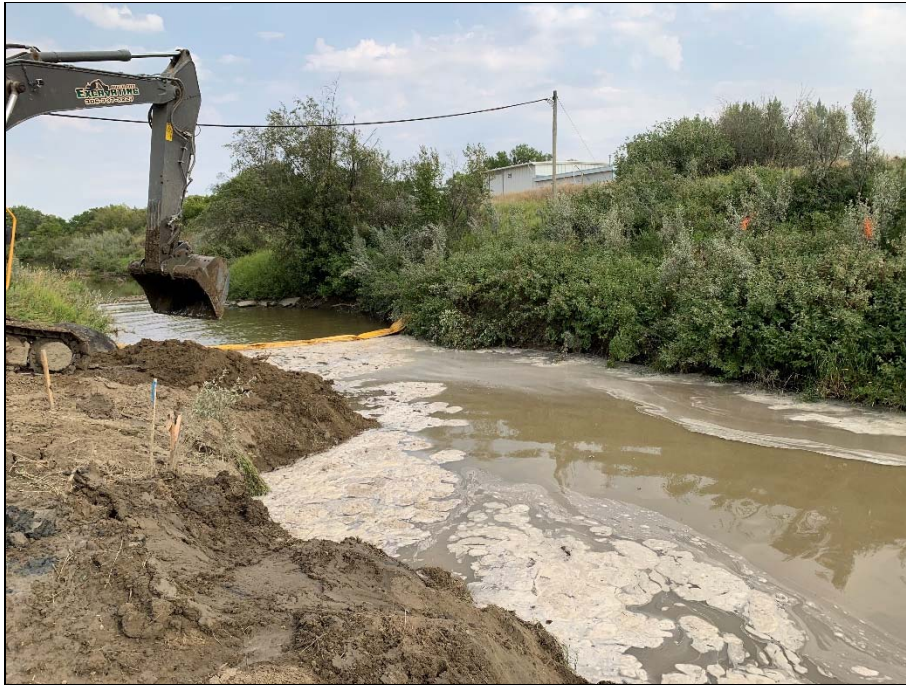
Removal of cofferdam and material from river bottom.
