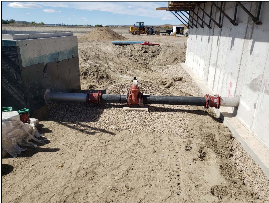
Connection between reservoir intake pumphouse and water treatment plant.
