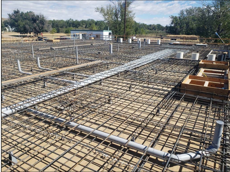
Top slab rebar and drainage piping inspection.
