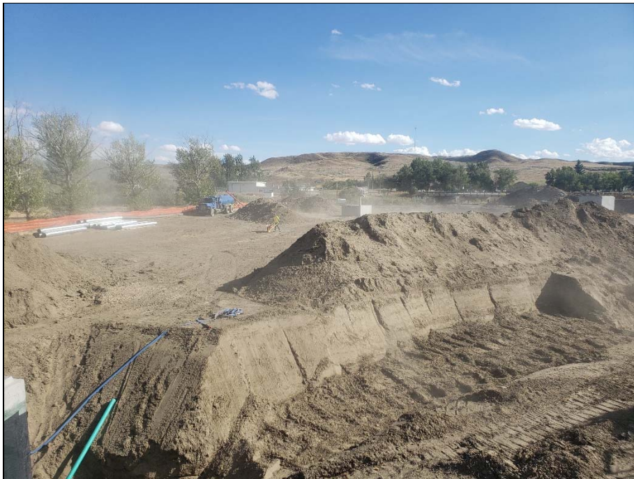
Excavation and earth moving from reservoir intake and pumphouse.
