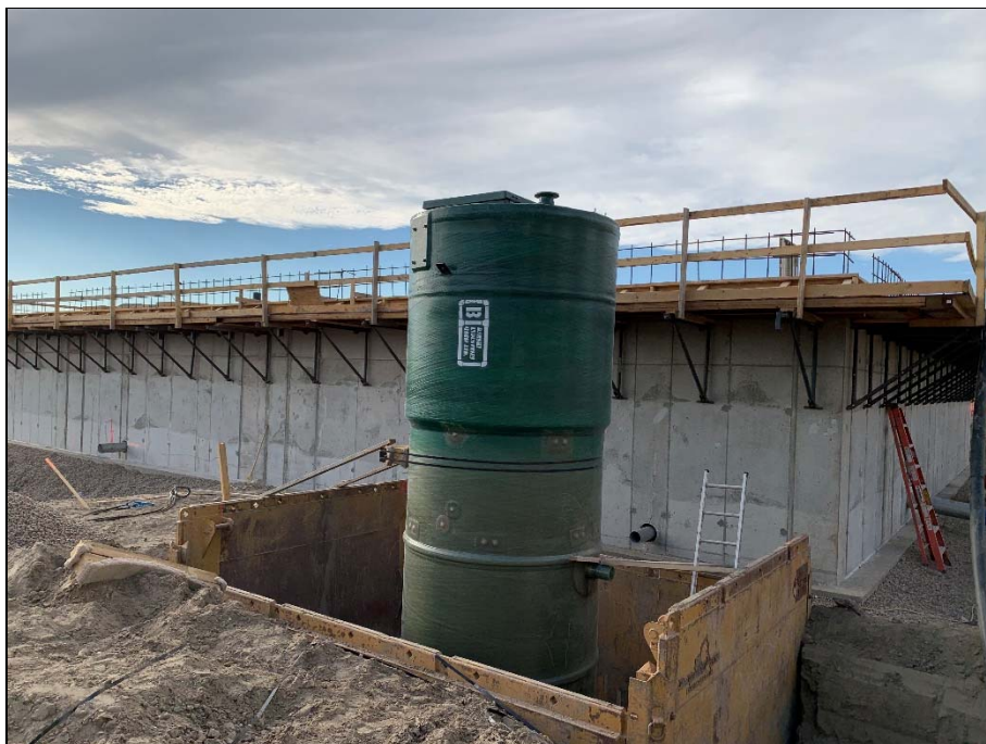
Effluent pumping station installation.
