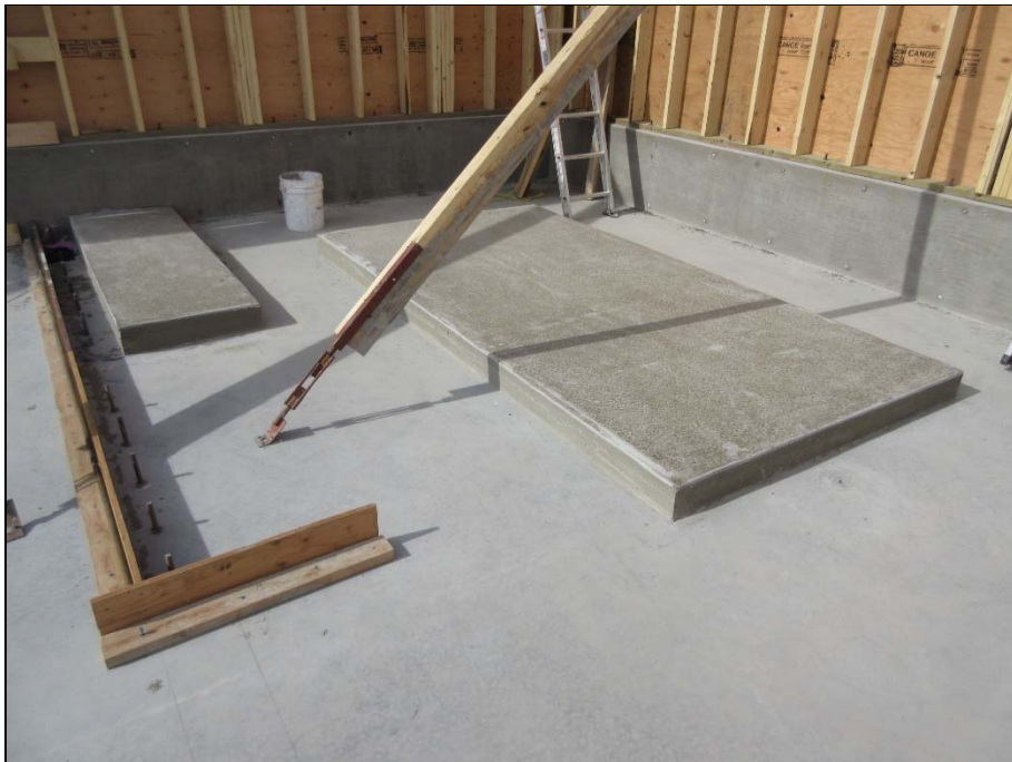
Generator set and air compressor equipment pads.
