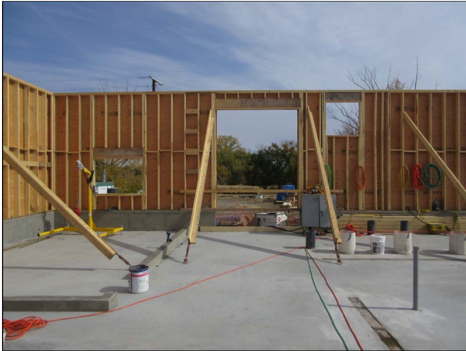
Exterior walls and door, window and louvre openings framed in.
