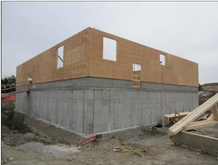
Exterior framing and sheathing is completed; truss construction at right.
