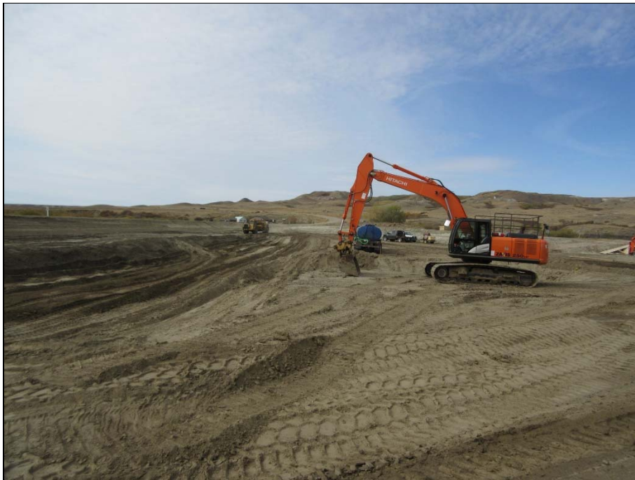
Earth moving from bottom of pond to build up berms.
